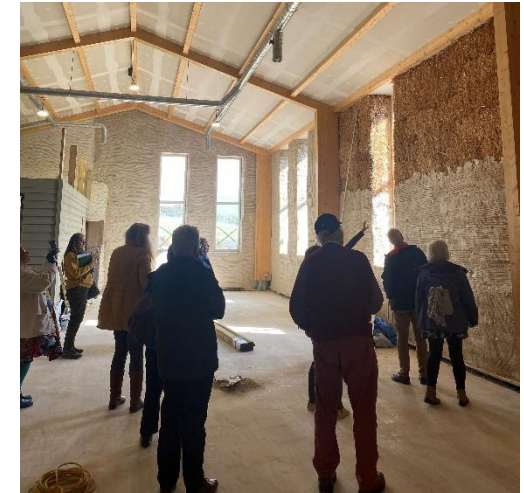
Image 5 Green Grid members at Elvis & Kresse, viewing the hay bale insulation of the new workshop
